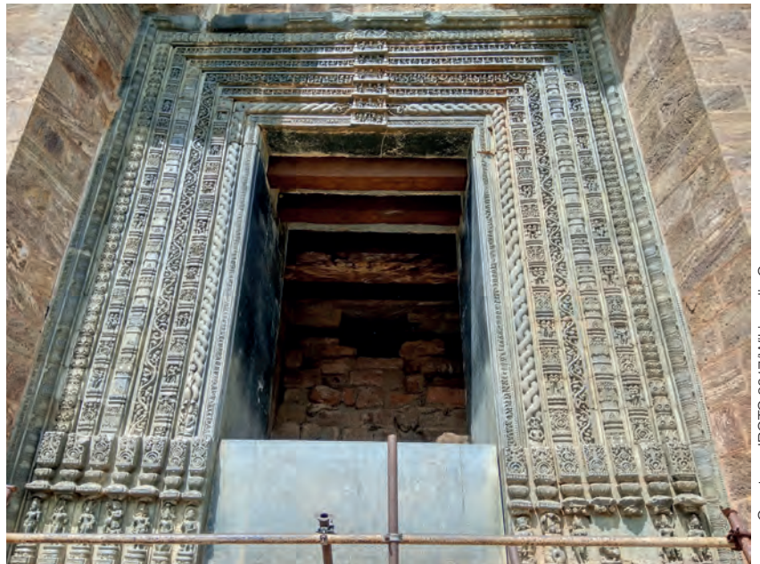
The marvellous entrance to the Sun Temple in Konark, carved in granite. Its non-rusting iron beams have withstood the test of time since the 13th century
