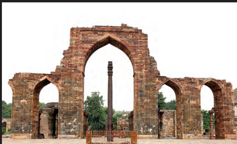
The 4th century iron pillar of Delhi is world renowned for its non-rusting property
